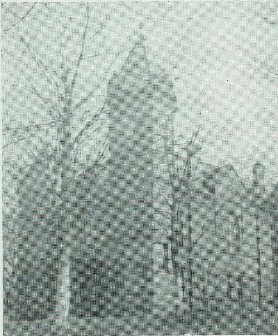
(No. 10 in a series of 55 front covers being used to present the Court Houses of West Virginia)
